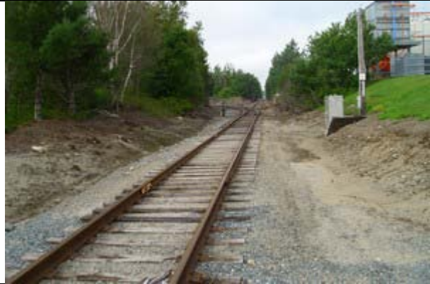
Tracks going into junction – sidings ahead
