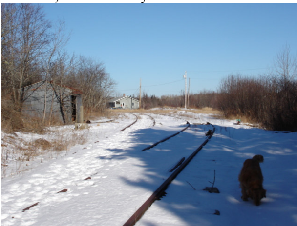
Looking east along toward Factory Road.
