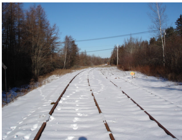
Looking east toward Route 191 along siding.
